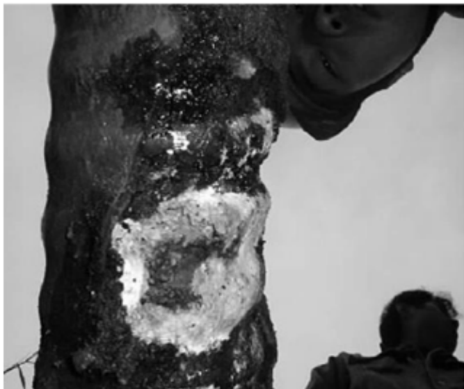
Figure 5: Cables eroded by white ants
