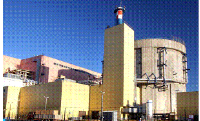
Figure 2: Cernavoda Unit 2, Reactor Building, Heavy Water Upgrader and Turbine Building (Right to Left)
