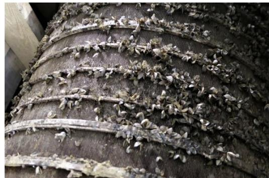
*Figure 1: Water inlet filter screen in hydropower colonized with Zebra mussels.*
